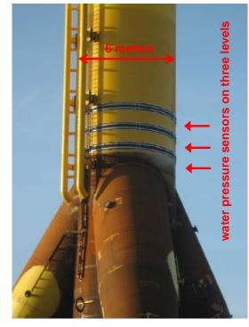
Fig. 1 Multibrid Tripod with measurement system (source: DEWI)
